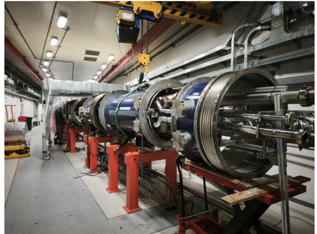
Figure 1. Installation of the last magnet of the NICA Collider.
