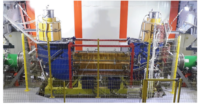
Figure 16. NICA Booster ECS installed in straight section of the synchrotron.
