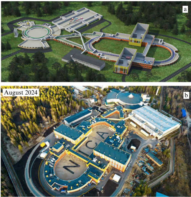
Figure 32. General views of NICA research complex with its main structural sites.
