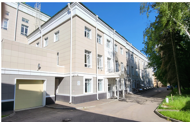
Building of the Center for High-Temperature Superconductivity (HTSC) and Quantum Materials, created on the initiative of V L Ginzburg (LPI RAS)
