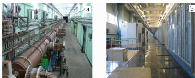
Photo 8. Accelerating cavities (a) and RF power gallery (b) of the main (600 MeV) segment of the accelerator.
