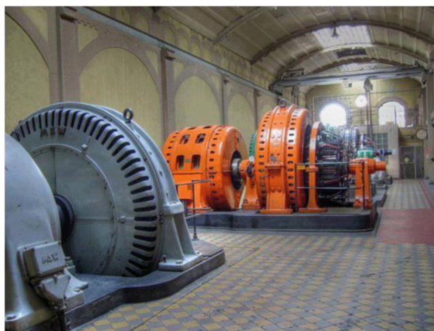
Figure 2. Motor-generator room for feeding the Bitter solenoids in the IL old building (current look).
