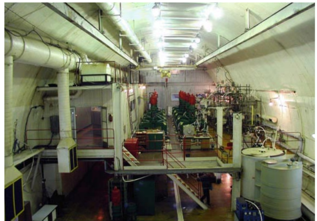
Figure 4. General view of the GGNT reactor hall.
