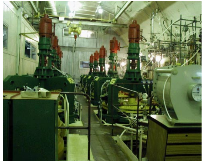
Figure 3. GGNT chemical reactors.
